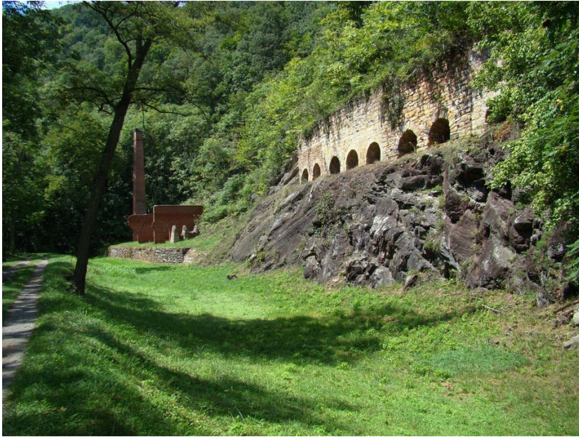
Remains of Roundtop Cement Mill near Hancock, MD On C&O Canal Path
